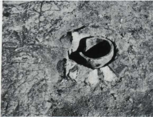
FIG. 234 - PALACE OF PHAISTOS - ROOM 69 a MODERN REPLICA OF ANCIENT CATCH-BASIN SET BELOW FLOOR LEVEL
