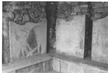
180 - HAGIA TRIADHA - BENCH, PARTLY RESTORED DADO, AND SOCKETS FOR VERTICAL BEAMS IN ROOM 4 (CF. FIG. 83).
