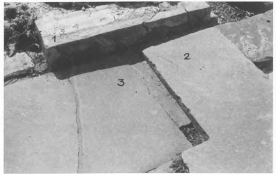
5 – PALACE OF MALIA - NORTHWEST ENTRANCE - DETAIL OF CUT JAMB-BASE OF SERPENTINE (1), SIDEROPETRA THRESHOLD BLOCK (2) AND PAVING SLAB (3).
