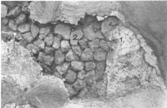
254 — MALIA - HYPOSTYLE CRYPT - FINE LIME PLASTER (1) APPLIED ON BACKING OF SMALL STONES (2).
