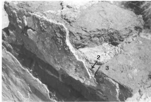
256 — PALACE OF MALIA - CORRIDOR C-C' - DETAIL OF WALL SHOWING LIME PLASTER (1), MUD PLASTER BACKING (2) AND MUD BRICK (3) IN BLOCKED DOORWAY.
