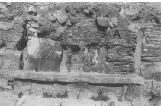
83 – PALACE OF KNOSSOS - WEST WING - REUSED GYPSUM SLABS IN WALL (BEHIND BENCH) IN THE LOBBY OF THE STONE SEAT.
