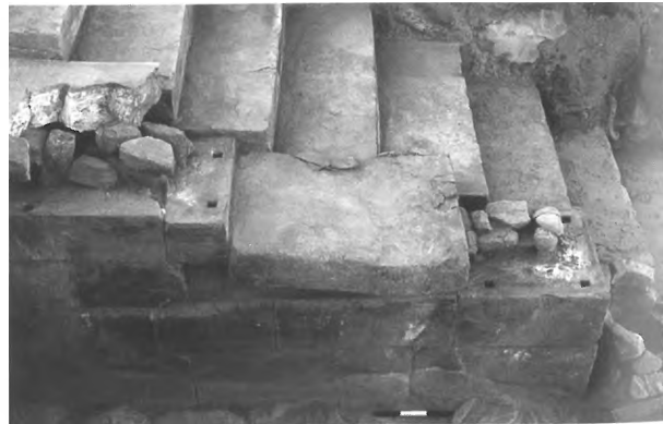
211B - MYRTOS-PYRGOS STAIRWAY, SHOWING DETAILS OF PIER BASES ALONGSIDE PARAPET.
