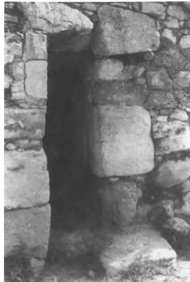
82 – PALACE OF KNOSSOS - SOUTH WING - REUSED LIMESTONE BLOCKS IN BASEMENT WALL.
