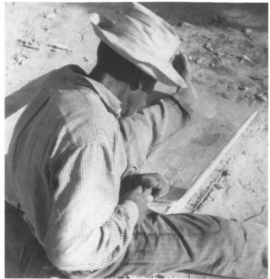
58B - HAGIA TRIADHA - A WORKMAN TRIMS A GYPSUM SLAB WITH A HAND-SAW - STEEL SAW-BLADE IS TOOTHED (SEE ALSO FIG. 58A).
