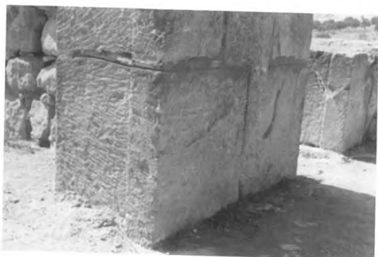
62A - PALACE OF PHAISTOS - MAGAZINE 29. JAMB WITH CHISEL MARKS.
