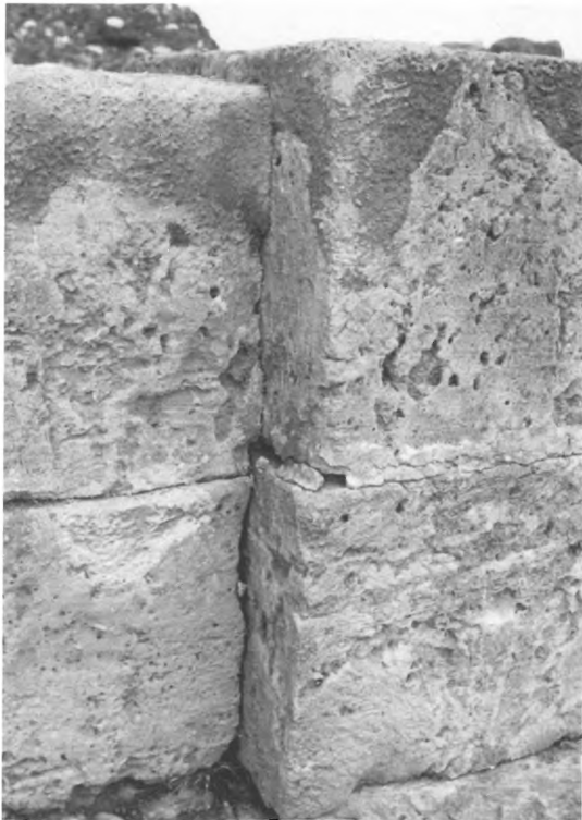
119 – PALACE OF MALIA - SET-BACK ALONG FAÇADE IN FIG. 118 - NOTE PLASTERED JOINTS.
