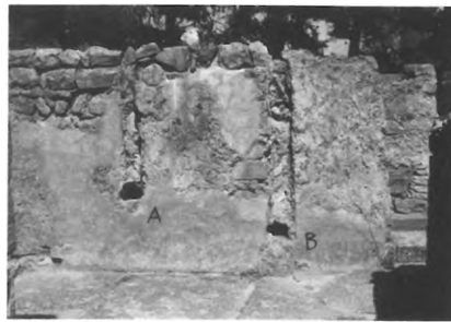
178 - TYLISSOS - HOUSE A. FORMS OF WOODEN PROPS IN EASTERN WALL OF ROOM 3. NOTE CAVITIES FOR HORIZONTAL STRUTS (SEE ALSO FIG. 179).
