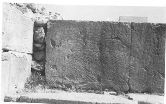
62B - PALACE OF PHAISTOS - CENTRAL COURT - WALL-BLOCK IN SECOND COURSE IN NORTHWESTERN CORNER - NOTE TOOL MARKS (FOR TOP OF BLOCK, SEE FIG. 221).
