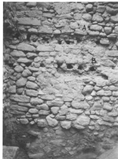
72 - FIRST PALACE OF PHAISTOS - BEAM SOCKETS IN WESTERN WALL OF ROOM IL.
