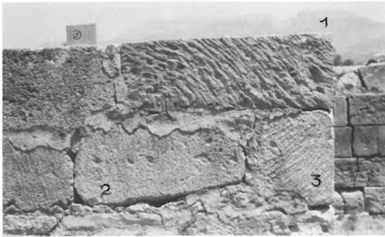
50 – HAGIA TRIADHA - DETAIL OF MODERN (RECONSTRUCTED) WALL OF BLOCKS OF POROS LIMESTONE NEAR «POTTER'S WORKSHOP», SHOWING MARKS OF MINOAN PICK OR CHISEL (AT 1), SMOOTHED MINOAN BLOCKS (AT 2) AND BLOCK CUT BY POST-MINOAN (MODERN?) TOOTHED CHISEL (AT 3).
