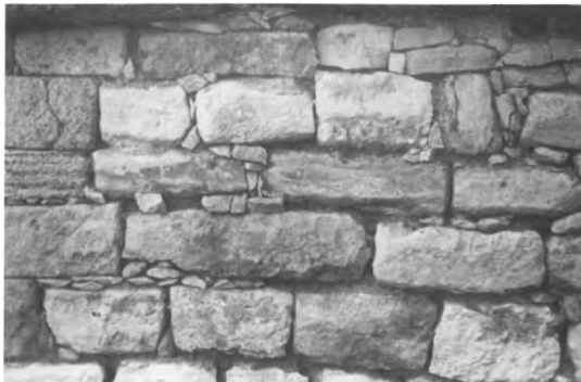
71 - PALACE OF KNOSSOS - DETAIL OF PLATFORM RETAINING WALL ALONG NORTHWESTERN BORDER.
