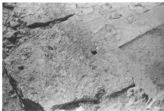
221 - PALACE OF PHAISTOS - TOP OF WALL ALONG NORTH-WESTERN SIDE OF CENTRAL COURT - NOTE BEAM BEDDING AND MORTISES (SEE ALSO FIGS. 62 B AND 216 [G]).
