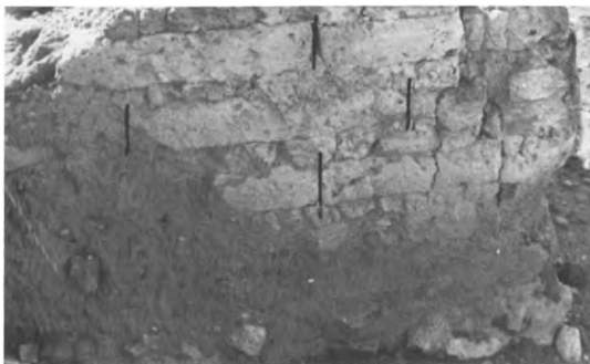
231 - PALACE OF KATO ZAKRO - WALL A IN FIG. 230. VERTICAL INKED LINES INDICATE JOINTS BETWEEN SEPARATE BRICKS.
