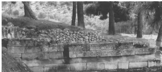
125a – HAGIA TRIADHA - LM III SHRINE (H) WITH PORTION OF ASHLAR WALL SET UPON HORIZONTAL TIMBER (NOTE CEMENT-FILLED CHASE ABOVE ASHLAR BASE COURSE. NOTE CHASE FOR VERTICAL TIMBER AT CENTER, LEFT) (LOOKING SOUTH) (SEE ALSO FIG. 188).
