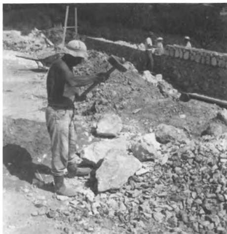
54 – KNOSSOS - WORKMAN BREAKING UP BLOCKS OF POROS LIMESTONE WITH A SLEDGEHAMMER.
