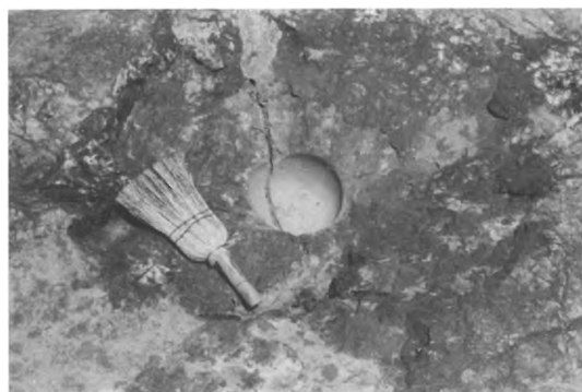
144B - PALACE OF PHAISTOS - DETAIL OF MORTISE FOR DOWEL IN FIG. 144 A.
