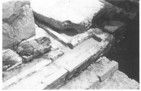
162B - PALACE OF KNOSSOS - TURN IN COURSE OF DRAIN IN FIG. 162A.
