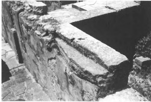
195A - TYLISSOS - HOUSE C - MORTISE FOR CLAMP (ARROW) AND BEDDING FOR BEAM CUT IN WALL-BLOCK, ROOM 15 (LOOKING SOUTHWEST).
