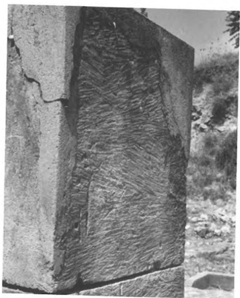
62C - KNOSSOS - LITTLE PALACE - PILLAR-BLOCKS WITH UPPER CORNERS RESTORED IN CEMENT. NOTE TOOL MARKS.
