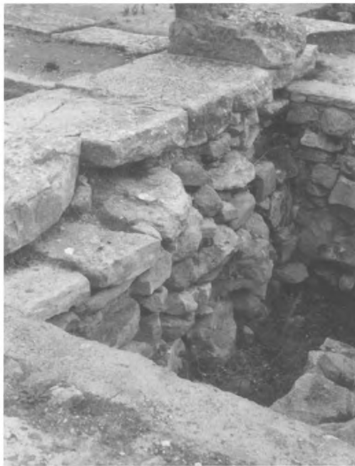
153 - PALACE OF PHAISTOS - STYLOBATE AND ITS FOUNDATION ALONG WESTERN SIDE OF CENTRAL COURT.
