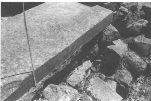
57B — TYLISSOS — HOUSE C, ROOM 10 — SQUARED THRESHOLD SLAB OF HARD GRAY LIMESTONE.
