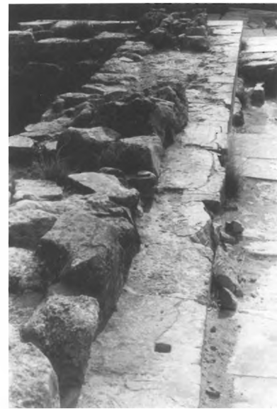
125b – HAGIA TRIADHA - LM III BUILDING ABCD (THE «MEGARON») SHOWING MORTISED ASHLAR BASE COURSE TO WHICH WOODEN BEAMS WERE DOWELLED (LOOKING EAST ALONG SOUTHERN WALL).
