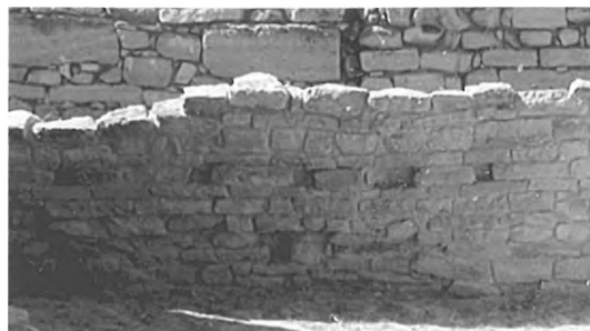
84 – KOMMOS - LOOKING SOUTH AT SOUTHERN WALL OF SPACES 29/25B OF BUILDING T, SHOWING PROBABLE SOCKETS FOR WOODEN SCAFFOLDING.
