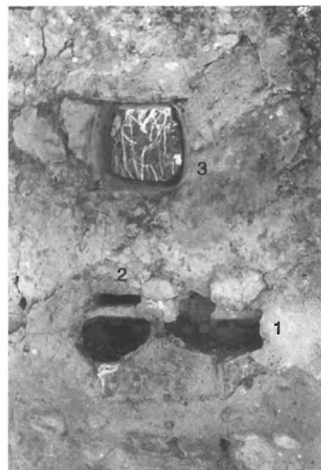
66 - VASILIKI - DETAIL OF WALL IN FIG. 65, SHOWING CAVITIES LEFT BY DISINTEGRATED TIMBERS (AT 1, 2) AND SMALL OPENING (WINDOW?) IN WALL (AT 3) (LOOKING SOUTH).
