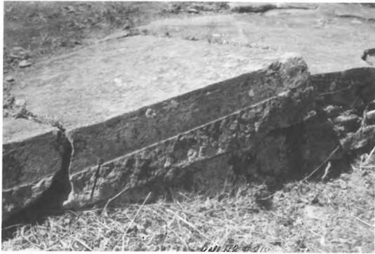
57D — HAGIA TRIADHA - SIDE OF SQUARED PAVING SLAB IN UPPER COURT - HARD GRAYISH-WHITE LIMESTONE. NOTE BOTTOM OF SAW-CUT.
