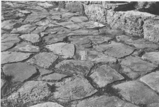
10 – NIROU KHANI - MAIN COURT, PAVING SLABS OF HARD LIMESTONE.
