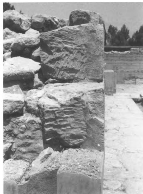
63C - PALACE OF PHAISTOS - WESTERN SIDE OF CORRIDOR 41 - ENDS OF WALL-BLOCKS SHOWING SMOOTHING OF JOINTS.
