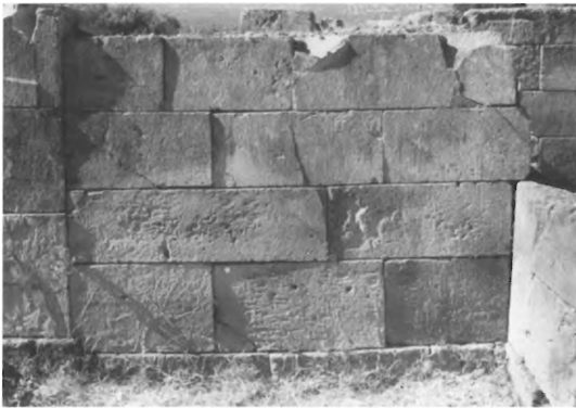
113 - HAGIA TRIADHA - BLOCKING WALL NEAR ROOM 1.
