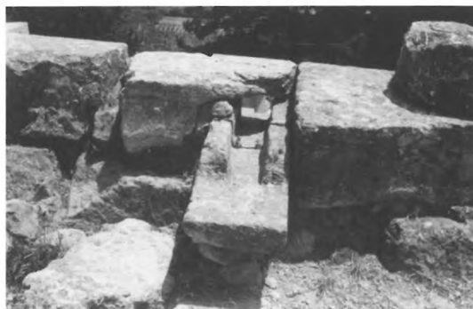
163 - PALACE OF KNOSSOS - COURT OF THE STONE SPOUT. END SECTION OF DRAIN LEADING TO THE COURT (LOOKING EAST) (SEE ALSO FIG. 101).
