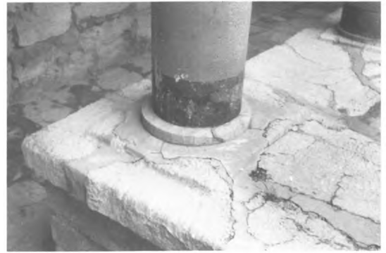
152 - PALACE OF KNOSSOS - PARAPET OF GRAND STAIRCASE WITH BASE AND COLUMN RESTORED.
