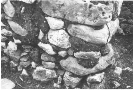
67 - GOURNIA - HOUSE AC - END OF A WALL BUILT OF MUD AND FIELDSTONES (BY AUTHOR).
