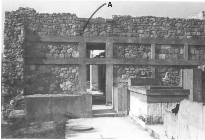
182A – PALACE OF KNOSSOS - RESTORED NORTH EXTERIOR WALL OF THE HALL OF THE DOUBLE AXES (BEAM BEDDING AT ARROW) (LOOKING SOUTH).
