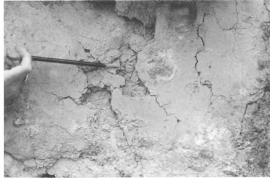
243 – VASILIKI - DETAIL OF WALL PLASTERING.
