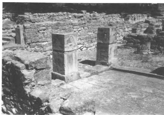
201 – TYLISSOS - HOUSE A - COMPLETE PILLARS BORDERING COURT IN ROOM 15 (LOOKING NORTHWEST).
