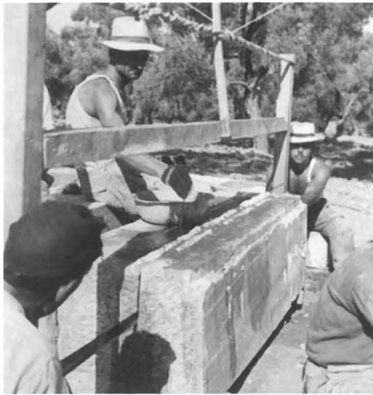
58A - HAGIA TRIADHA - CUTTING OF LARGE SLABS OF GYPSUM FOR MODERN RESTORATION WORK - THE SAW-FRAME IS PARTIALLY SUPPORTED BY ROPES; THE STEEL SAW IS TOOTHED. MAN IN CENTER ADDS WATER TO COOL THE BLADE AND TO REDUCE FRICTION.
