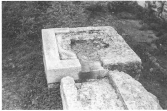
162A - PALACE OF KNOSSOS - BASEMENT OF EAST HALL. PARTIALLY RESTORED DRAIN HEAD AND WATER CHANNEL.
