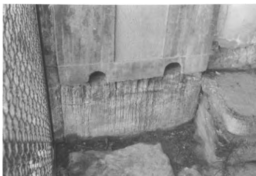
205 - PALACE OF PHAISTOS - BOTTOM OF PARTLY RESTORED PIER IN ROOM 50 - SEMI-CIRCULAR HOLES LEFT IN CONCRETE ALLOW ONE TO INSPECT MORTISE SOCKETS.
