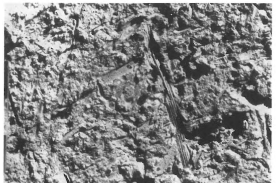
226 - TEXTURE OF MUD MORTAR - NOTE IMPRESSIONS OF DISINTEGRATED BINDING MATERIAL.
