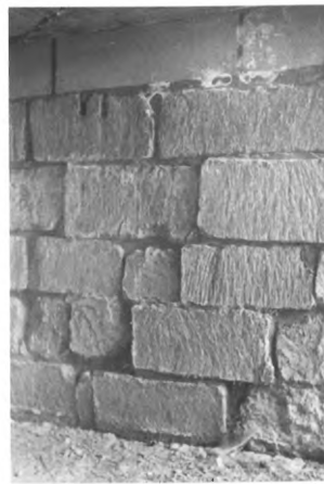
105 – KNOSSOS - EASTERN WALL IN BASEMENT OF SOUTH HOUSE.
