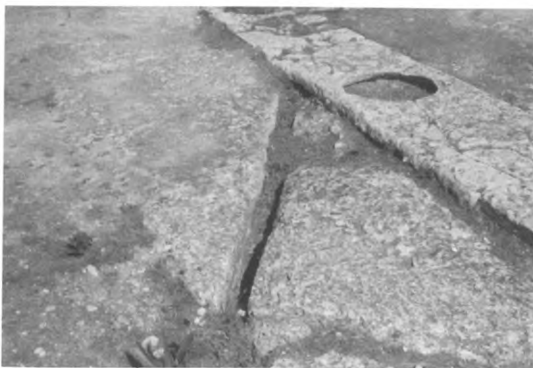
160 — PALACE OF PHAISTOS - DRAIN CUT IN BEDROCK NEAR COURT 64.
