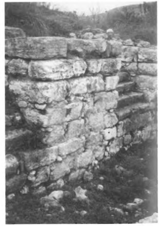
106 – KNOSSOS - VIADUCT (LOOKING NORTHWEST).
