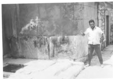
94 - PALACE OF KNOSSOS - ROUNDED CORNER IN NORTHWESTERN CORNER OF CENTRAL COURT. THE CONCRETE RESTORATION INDICATING COURSED ASHLAR MASONRY IS PROBABLY ERRONEOUS.
