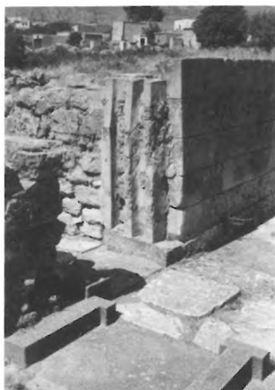
189 – TYLISSOS - HOUSE C - PARTLY RESTORED JAMB WITHOUT HORIZONTAL TIMBER.
