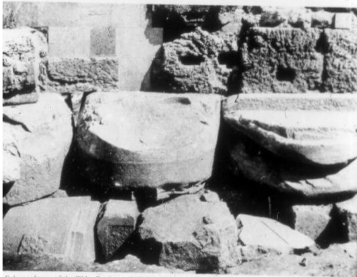
Column drums of the Older Parthenon built into the north wall of the Acropolis.
