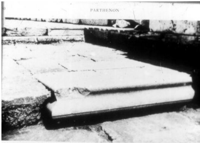
9 Anta base of the Older Parthenon, re-used in the foundations of the Parthenon floor.
