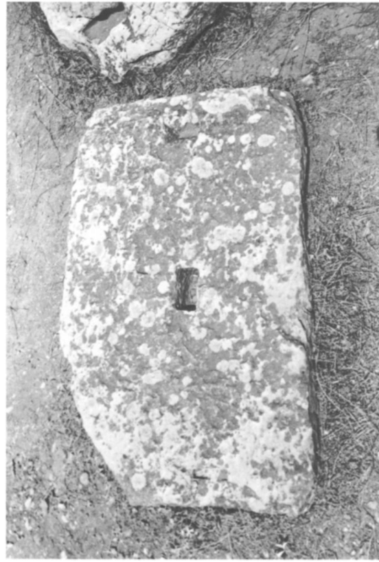
d. Top of front horizontal geison block G60 41A (Roman replacement)
