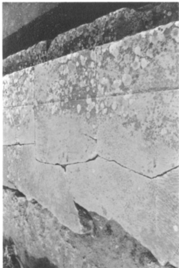
a. Top of the middle step, north side, showing polygonal joints, chisel marks, and pry holes
