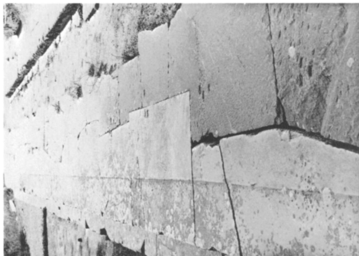
b. Middle step, north side, from the west, showing polygonal joints
