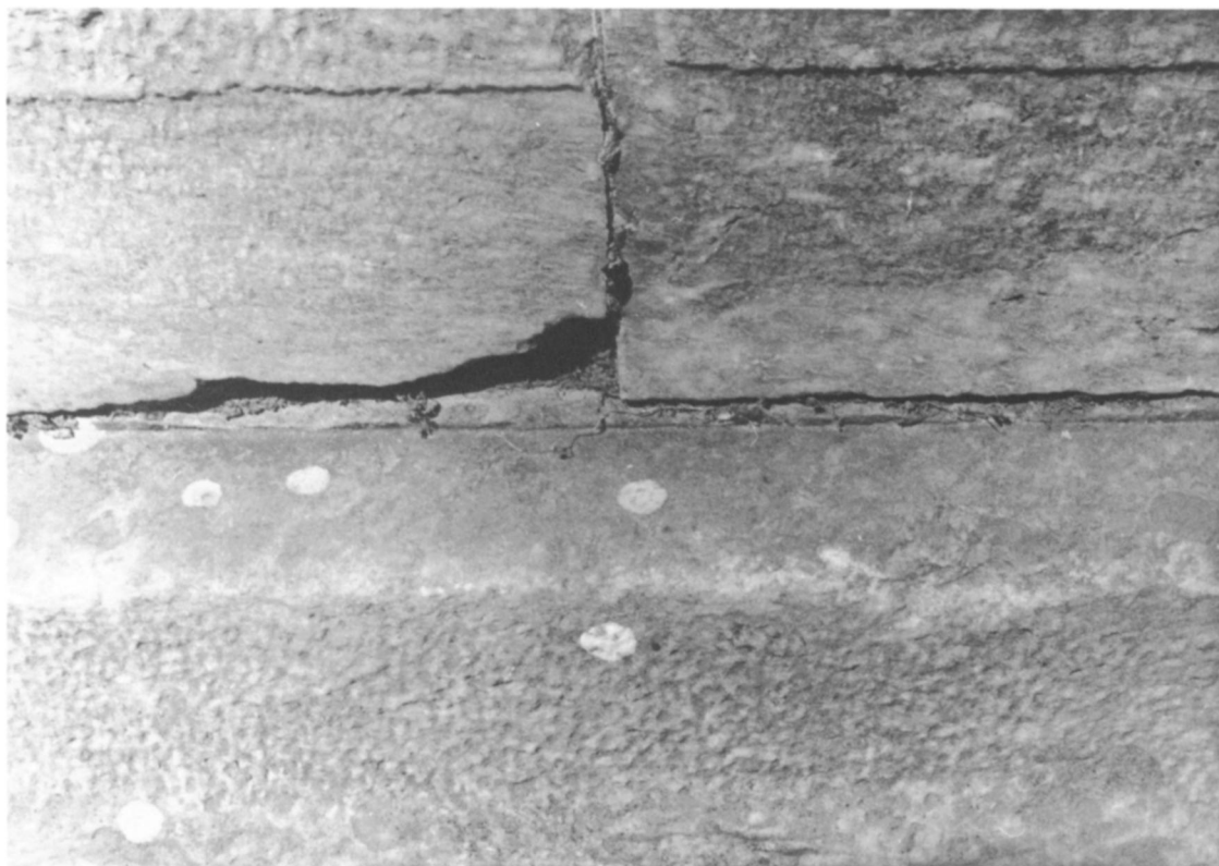
a. Raised ledge on the top of the euthyteria, east side
