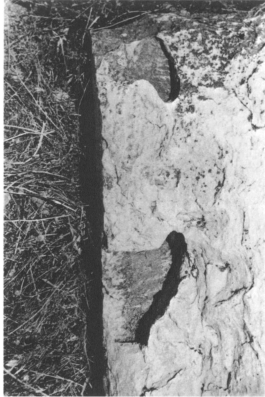
d. Cuttings for lifting tongs in the top of a fragmentary backer block
