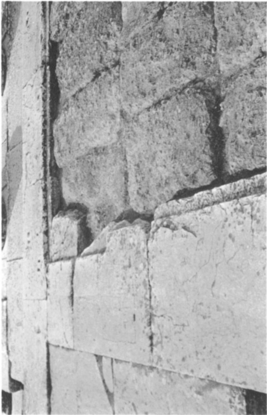
a. Conglomerate packing in the southeast corner of the cella
