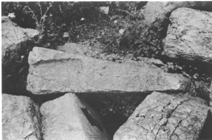
c. Temple of Apollo, Bassai: trapezoidal backer block to support the sima above the flank geison
