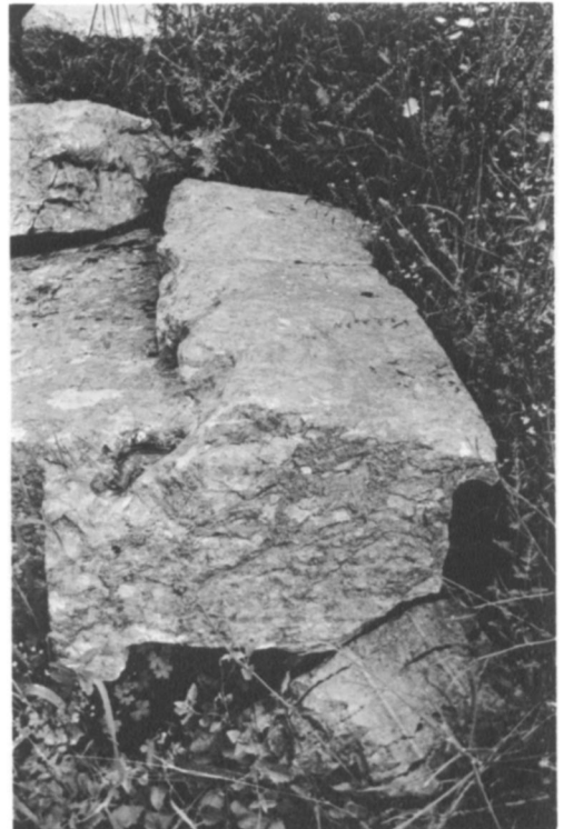
d. Temple of Apollo, Bassai: front of a flank geison block showing the inclined ledge to support the sima
