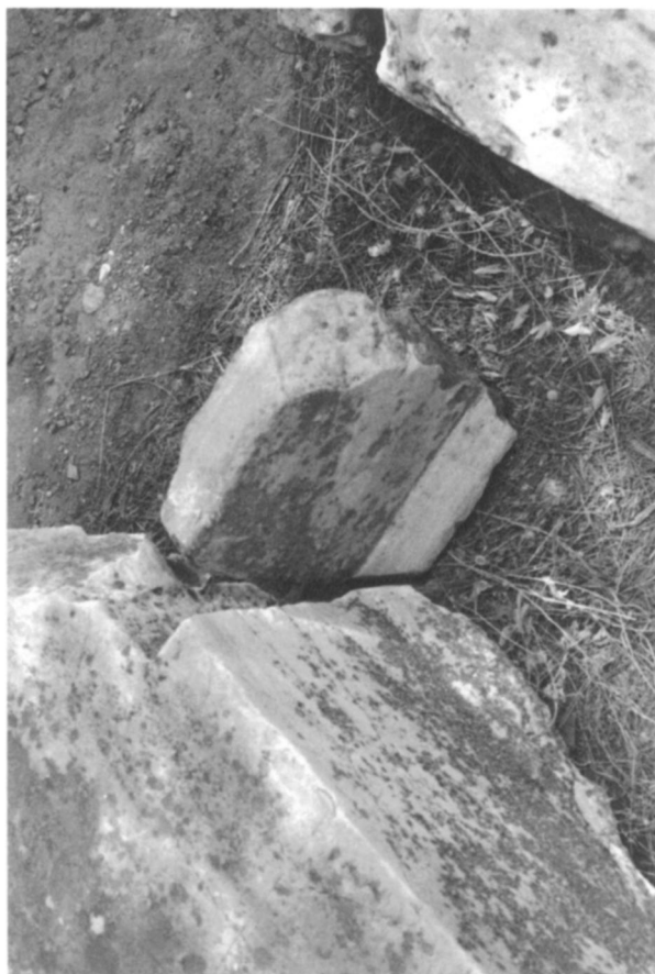
b. Fragment of a filler panel set into a beam slot (upside down)
