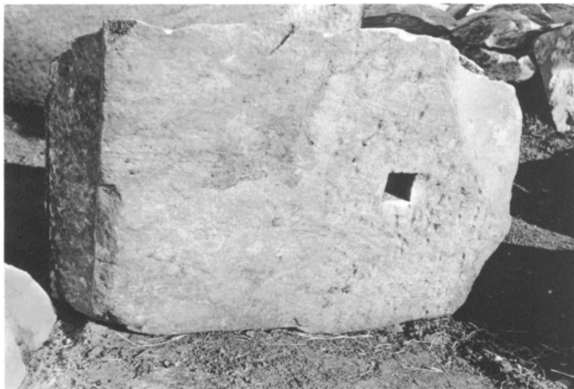
a. Bottom of the southwest corner sima block RT4 134D with a cutting for a blind dowel
