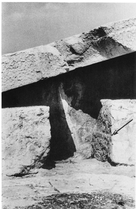
FIG. 17. Ledge in SW purlin cutting
