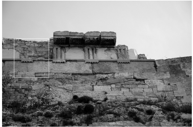
Fig. 3. Athens, temple of Athena Polias: entablature blocks reassembled and exposed in the northern fortification wall of the Acropolis (photo G. Rocco).
