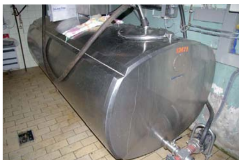
Fig. 4.2-14 Stainless-steel vessel for the storage of up to 2000 L of raw milk at a farm in the Swabian Mountains
