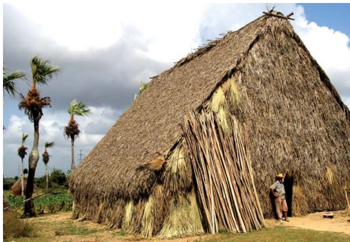
Fig. 1.1-12 A cottage made from eucalyptus stakes covered with palm fronds is the typical equipment for processing raw tobacco leaves in Cuba
