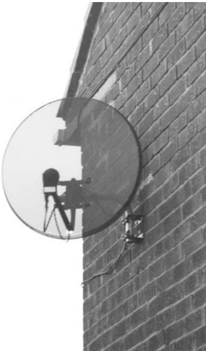
Figure 13.6 Offset metal mesh dish for satellite reception
