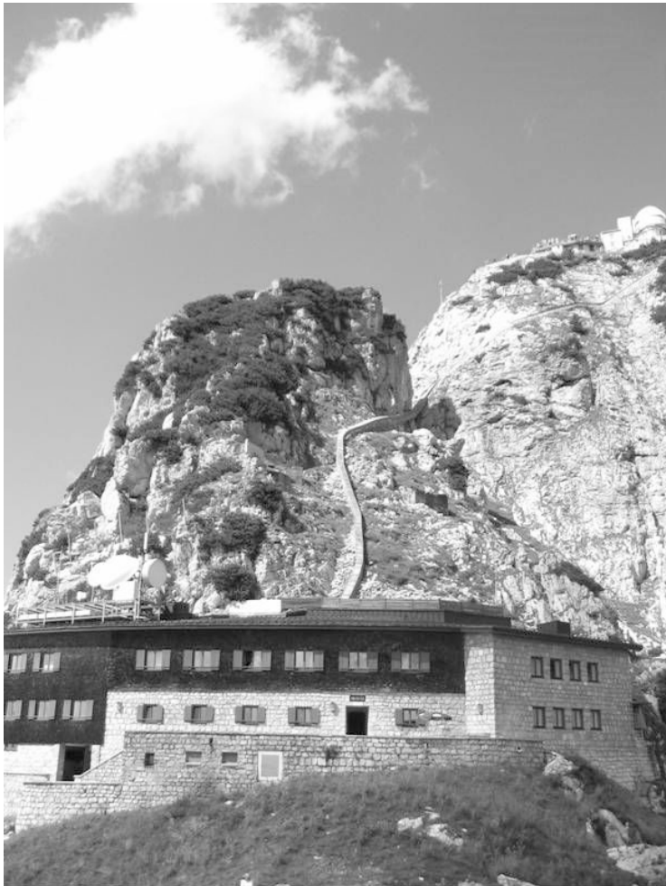
Fig. 46.3. Transmission station Wendelstein, Bayerischer Rundfunk, directional radio antennas and cable duct for the transmission cable clearly recognizable
