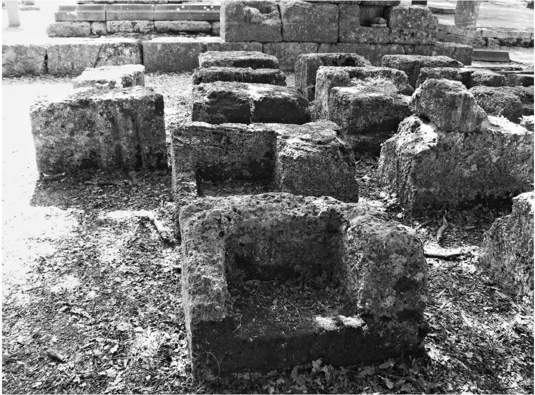
Figure 2. Triglyph-blocks from the Echo stoa at Olympia with roof-beam sockets.
