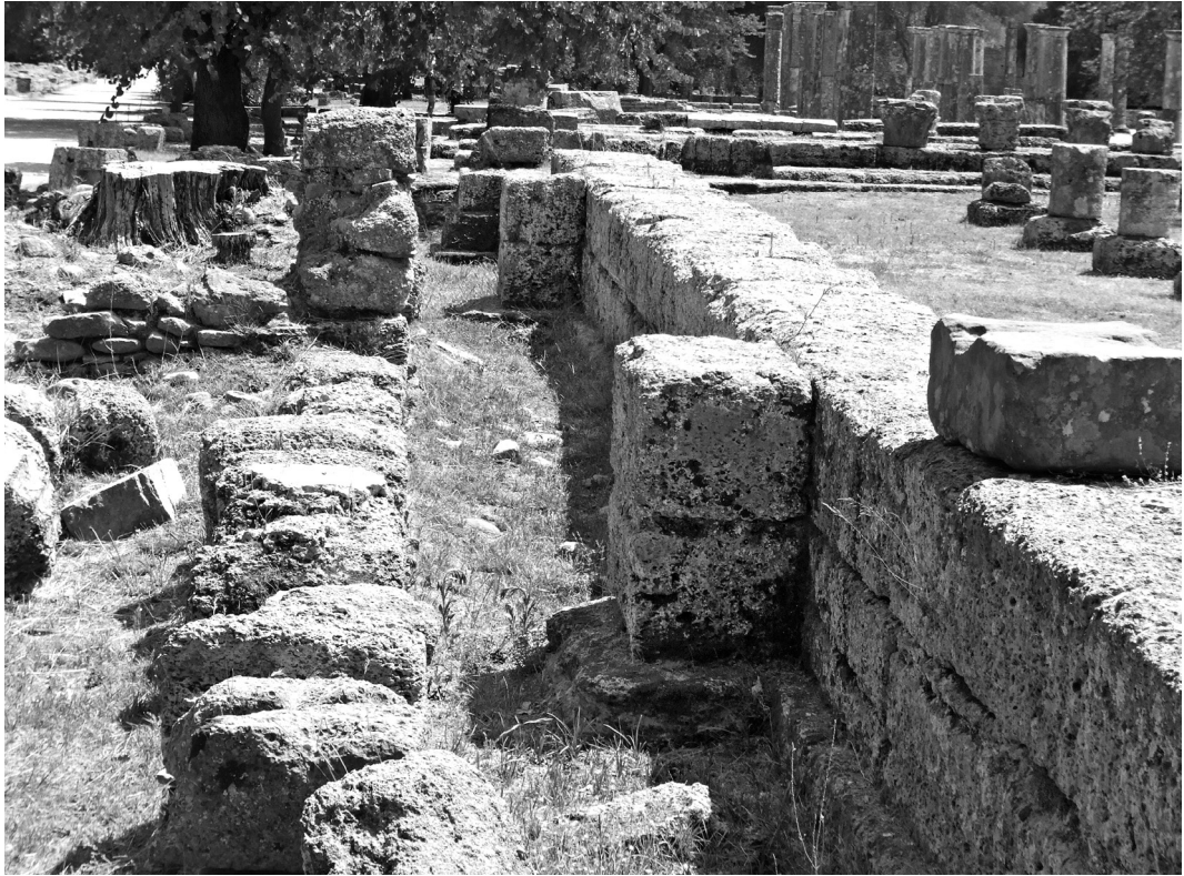
Figure 3. Buttressed toichobate of the Gymnasium east stoa at Olympia.
