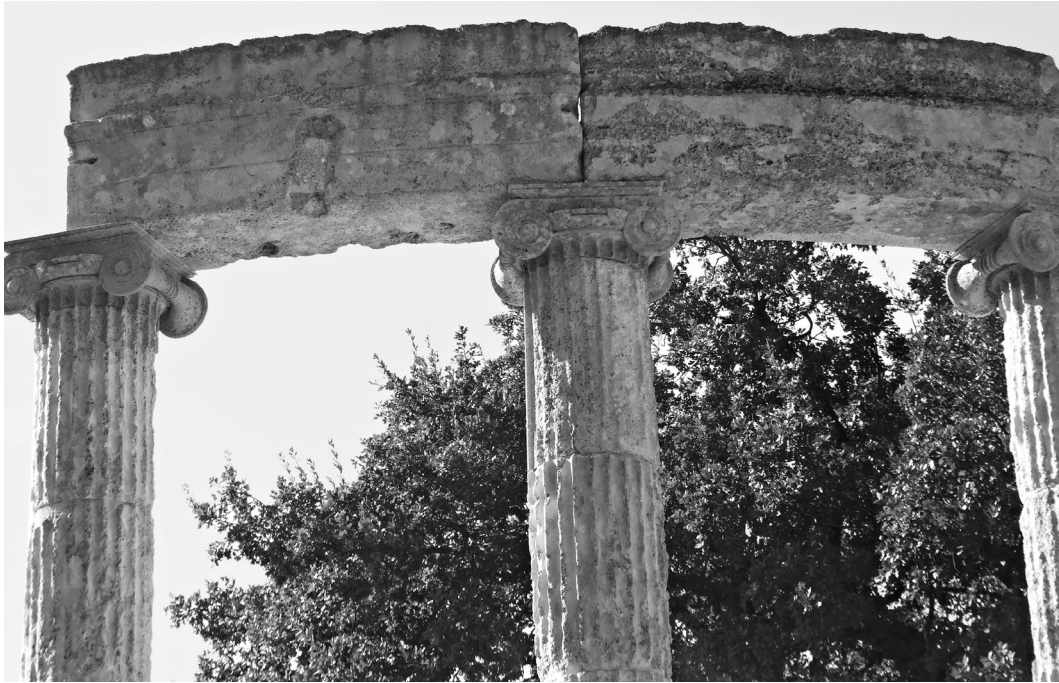
Figure 1. Part of the Philippeion epistyle at Olympia showing traces of repairs.
