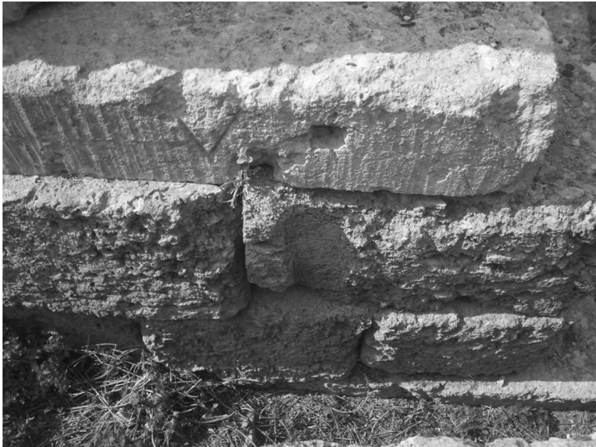
Fig. 15. Vertical cutting in euthyneria course.
