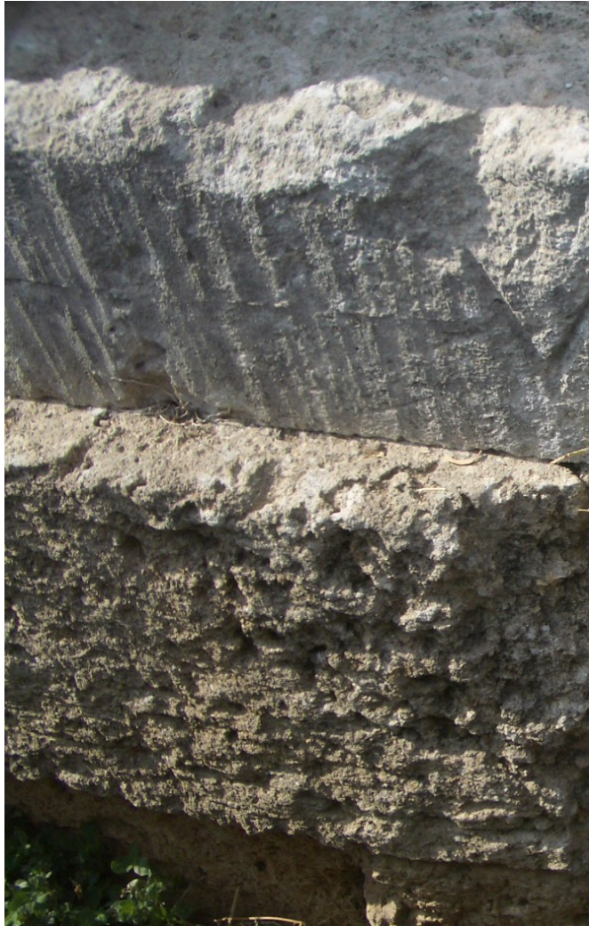
Fig. 11. Vertical tool marks left by flat chisel on inside face of krepidoma, showing difference in tooling between krepidoma and euthynteria course below.
