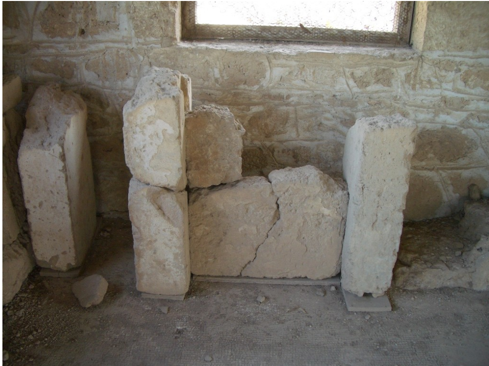
Figure 107. Preserved sections of piers and parapet slabs.
