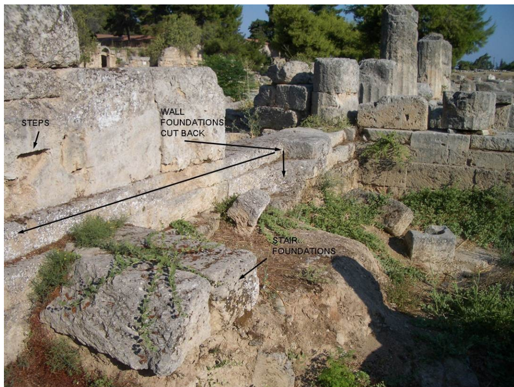
Fig. 18. West wall showing step cuttings. Toichobate cut back to accommodate original stair foundations.
