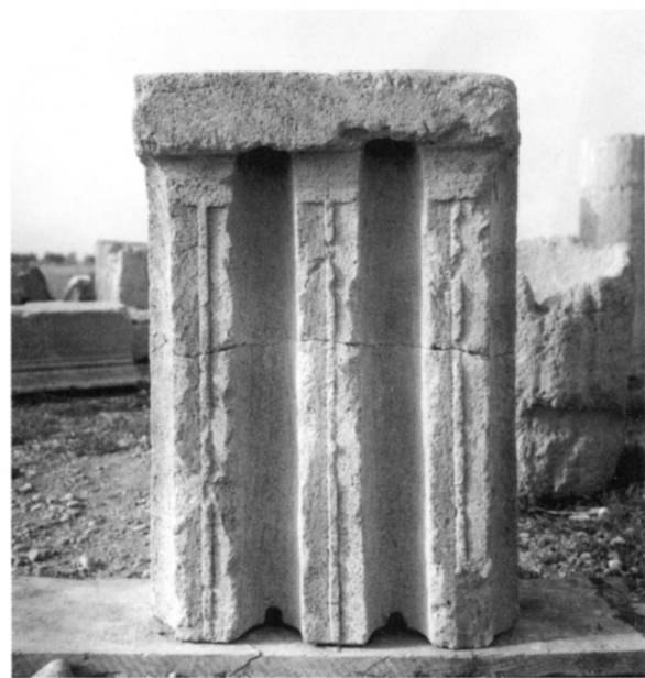
Fig. 24. Triglyph from the so-called Tavole Palatine, Metapontum, third quarter of the sixth century; note the rib on the front face of the glyph, the concave profile of the sides of the glyph and the slight gap between the glyphs. (Mertens 1993, Taf. 73.2)
