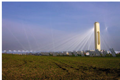
This solar power plant in Spain is using a large number of mirrors reflecting sunlight toward the top of the tall tower. The intense focused light heats up water, and the steam it produces is driving a turbine and generating enough energy for 6,000 homes (flickr/afloresm).
