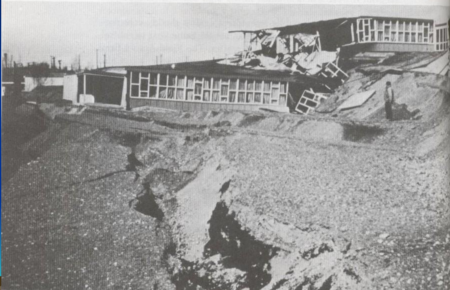
Figure 8 Wrecked modern school building in Government Hill slide area, Anchorage, Alaska (1964). The building withstood the shaking but not the landslide. The earthquake occurred during a school holiday. [Courtesy of USGS.]
