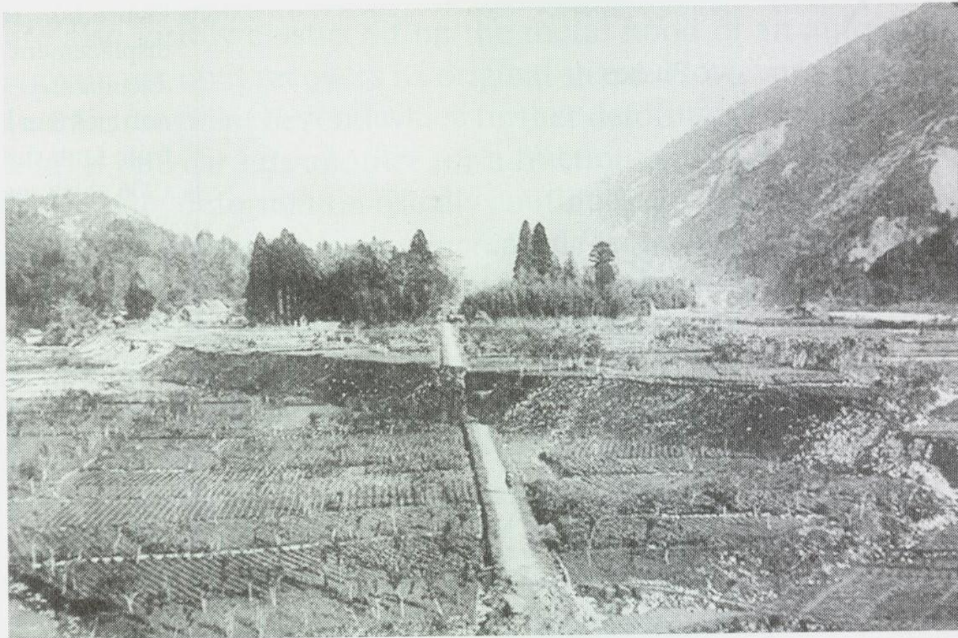
Figure 1.6 The Mino-Owari fault scarp that resulted from the 1891 Japanese earthquake. Notice the displacement of the road crossing the fault scarp.
