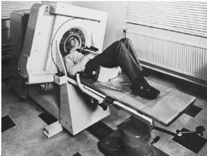
Fig. 3.5. The first head scanner was built in the EMI Central Research Laboratories in London. Courtesy of General Electric Medical Systems
