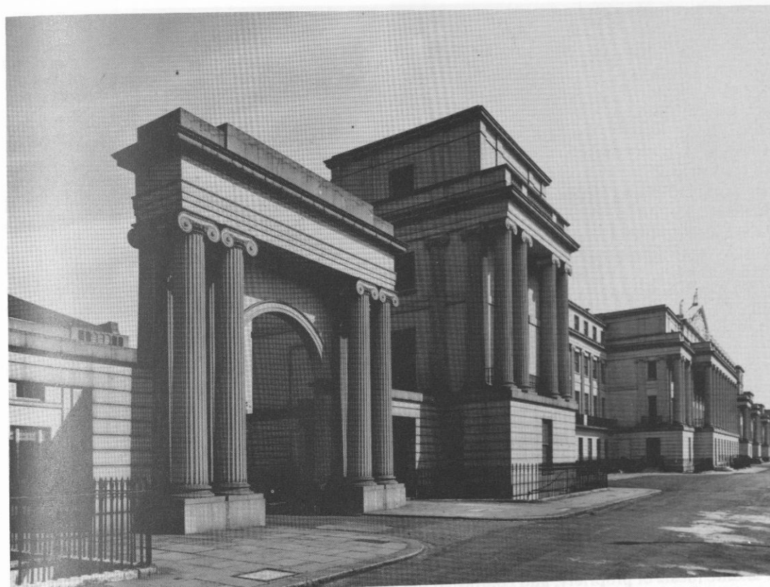
FIGURE 2. The masterpiece of Classical revival in London: John Nash, Cumberland Terrace, St Pancras, London, 1826, part of Nash's grand design for Regent's Park. As an architectural design it is 'among the most splendid of its day in Europe' (Pevsner 1952: 346), to be compared in scale only with what went up at the same time in St Petersburg, and a supreme exemplar of creative re-use of the Greek heritage though Roman rather than Greek. (Photo: RCHME.)
