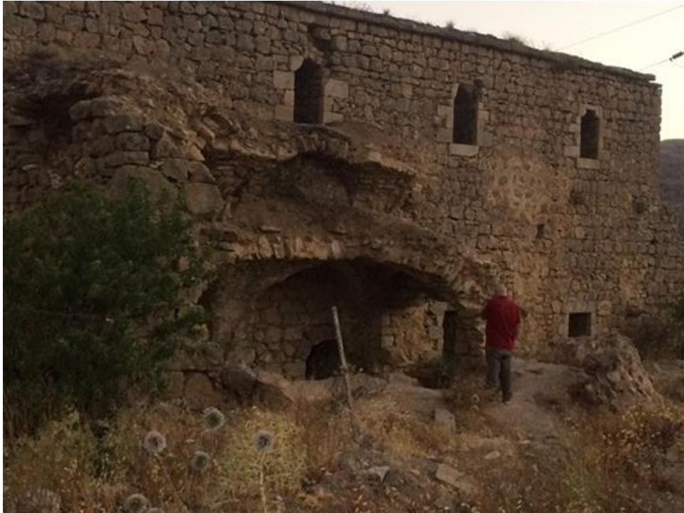
Church at Çüngüş village
