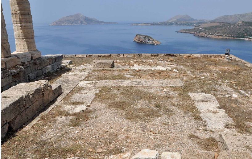
Figure 13. View of the interior of the Classical temple, with the foundations of the Archaic temple visible at center, from the east. Photo J. Paga
