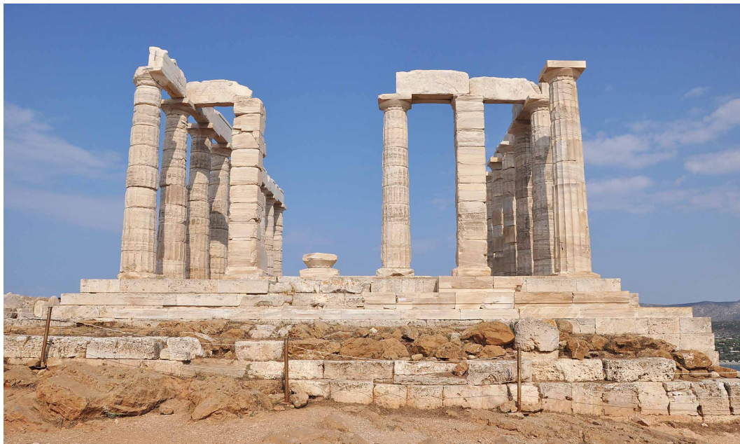
Figure 5 ( above ). View of the east supporting terrace and foundations of the Classical temple, showing reused blocks from the Archaic temple, from the east. Photo J. Paga
