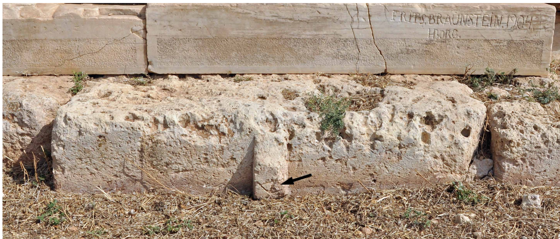
Figure 17. Step block (S3) with lifting boss bearing mason's mark—an upside-down "A"—embedded in the south flank beneath the marble euthynteria. Photo J. Paga
