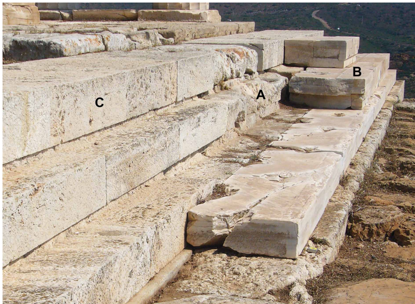
Figure 15. Steps along the eastern facade of the Classical temple, showing marble overlapping limestone blocks of the Archaic temple. A: Archaic limestone steps; B: Classical marble steps; C: modern replacement steps. Photo M. M. Miles
