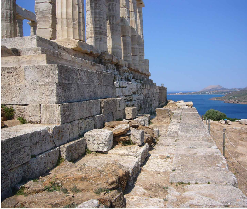
Figure 8. View along the north flank of the Classical temple, where much of the supporting terrace is robbed out. At center, traces remain of a post-antique cistern built through the supporting terrace. Photo M. M. Miles
