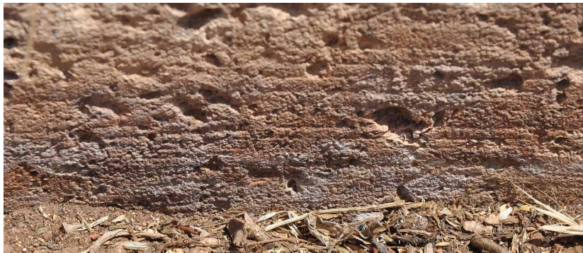
Figure 16. Detail of the vertical face of step block (S1) with possible traces of burning, embedded in the south flank beneath the marble euthynteria. Photo J. Paga
