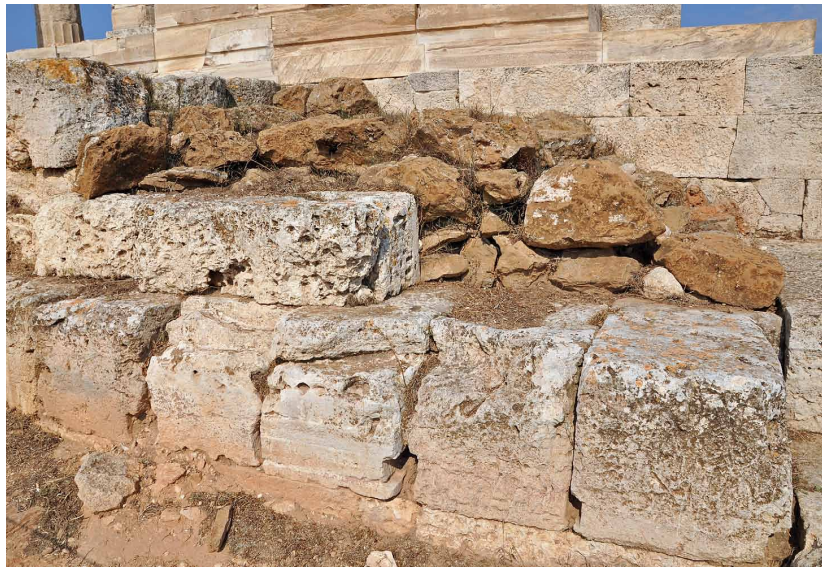
Figure 28. Triglyph blocks (T1–T6, right to left) built into the east supporting terrace. Photo J. Paga
